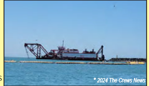
April 2024 - Manson dredger at harbor entrance.
