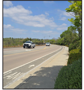
Southbound Douglas at Cardiff Bay Drive.
